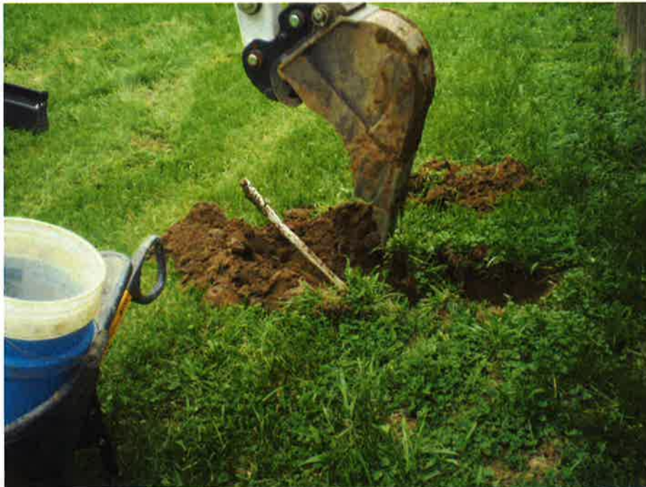
Photo 18. Casing pulled during excavation of MP-8E.
