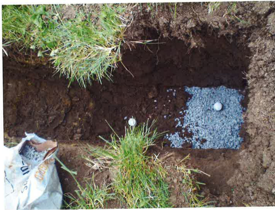
Photo 11. MP-7F and unknown probe have been capped and bentonite chip placement has started.
