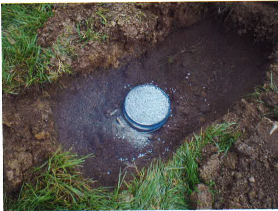
Photo 24. Bucket form filled with bentonite chips above MP-8R.
