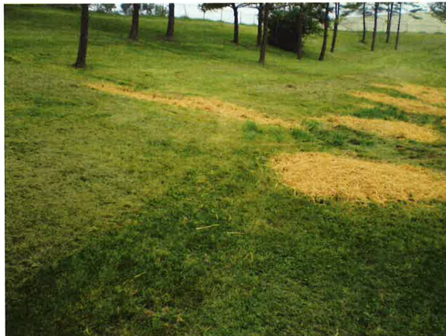
Photo 48. Some soil was added to the settled area in the vicinity of the vacuum break.
