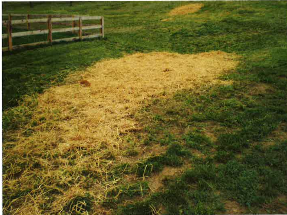
Photo 53. Soil stockpile area seeded and covered with straw.
