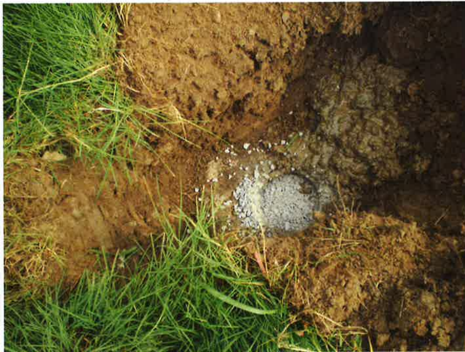
Photo 4. Bentonite chips placed in buried flush mount protective casing at SP-14.
