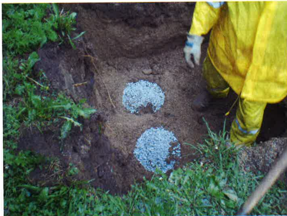
Photo 26. Bentonite chips placed above MP-8D and PPA.
