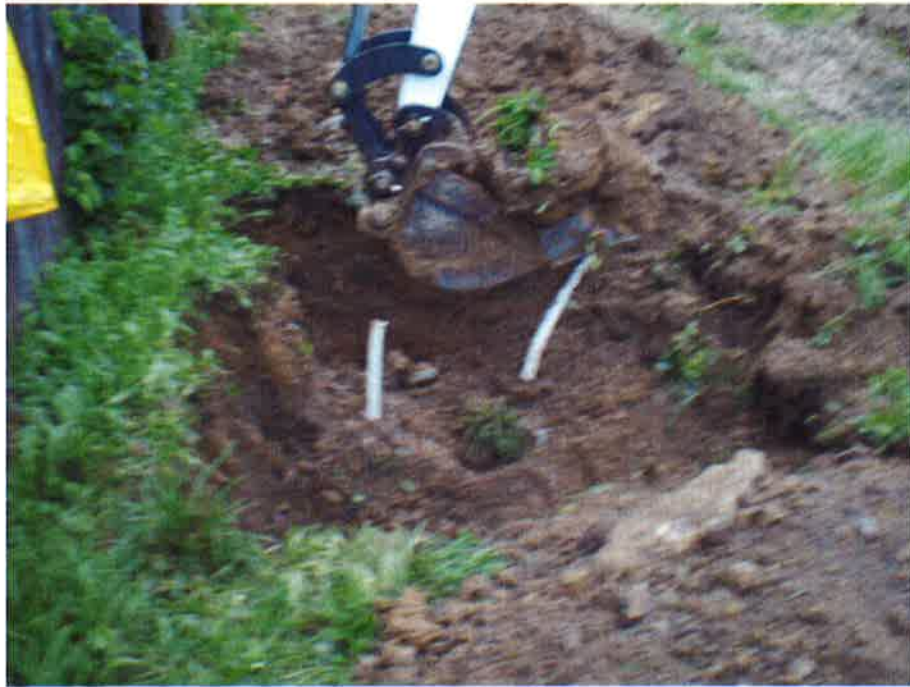
Photo 27. Excavation of DPC and FPC.
