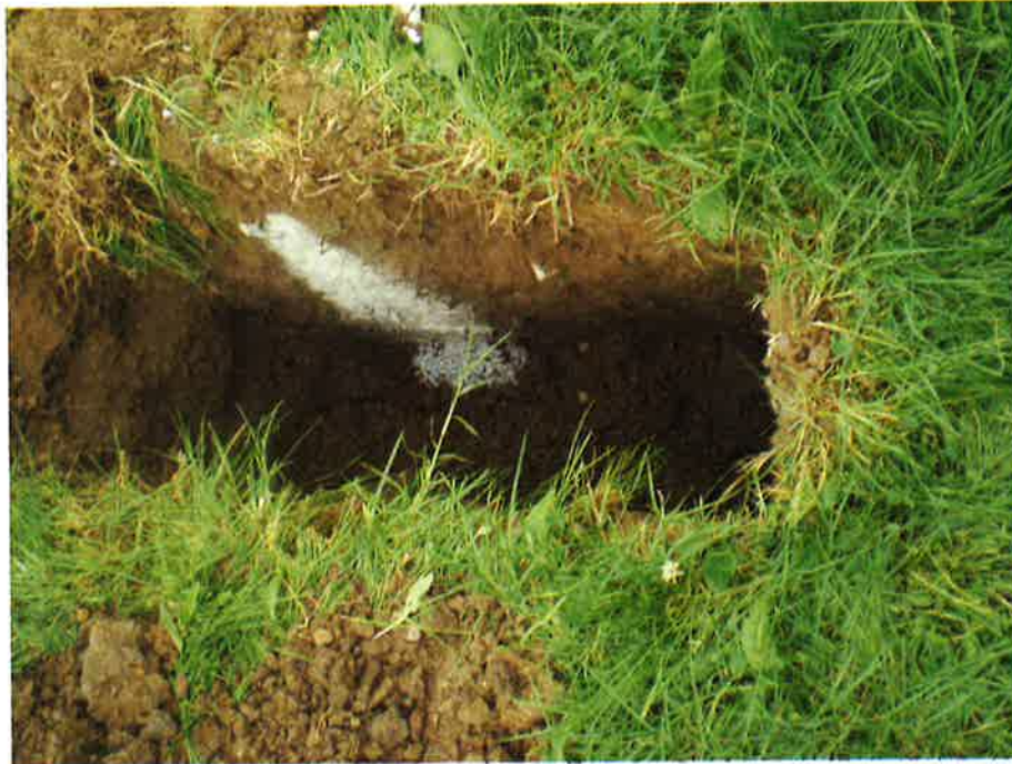
Photo 21. Placement of bentonite chips above MP-8AR using soil to contain chips.
