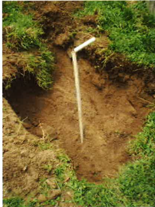
Photo 15. MP-8G casing pulled out of excavation.
