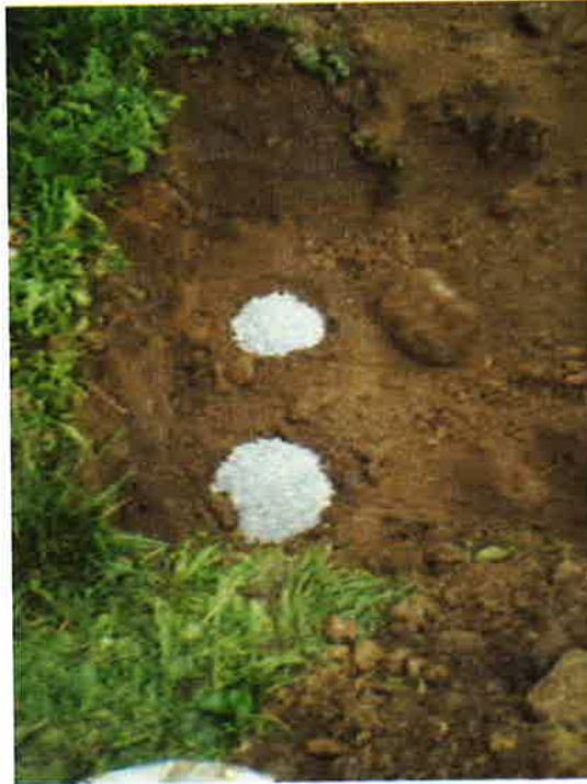
Photo 31. Bentonite chips placed above DPC and FPC.
