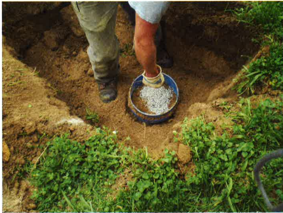
Photo 19. Removal of bucket form after backfilling around bucket, prior to hydration of bentonite chips at MP-8E location.
