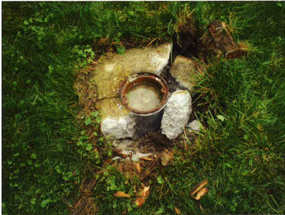
Photo 1. MP-15 with concrete pad partially removed.
