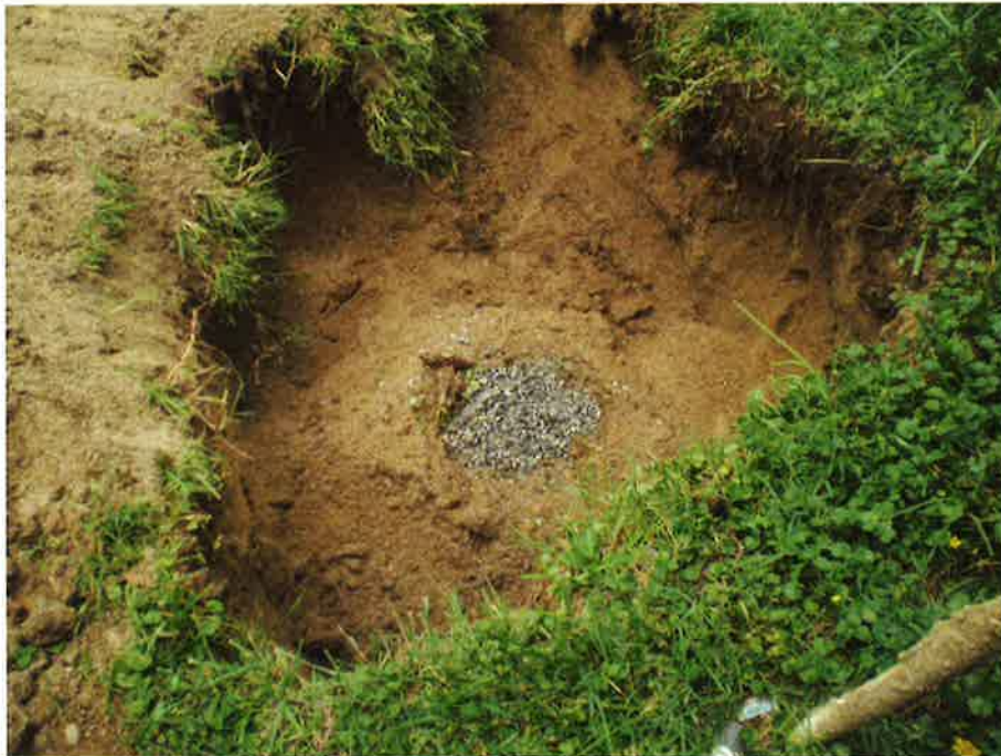
Photo 16. Bentonite chips placed above MP-8G and hydrated.
