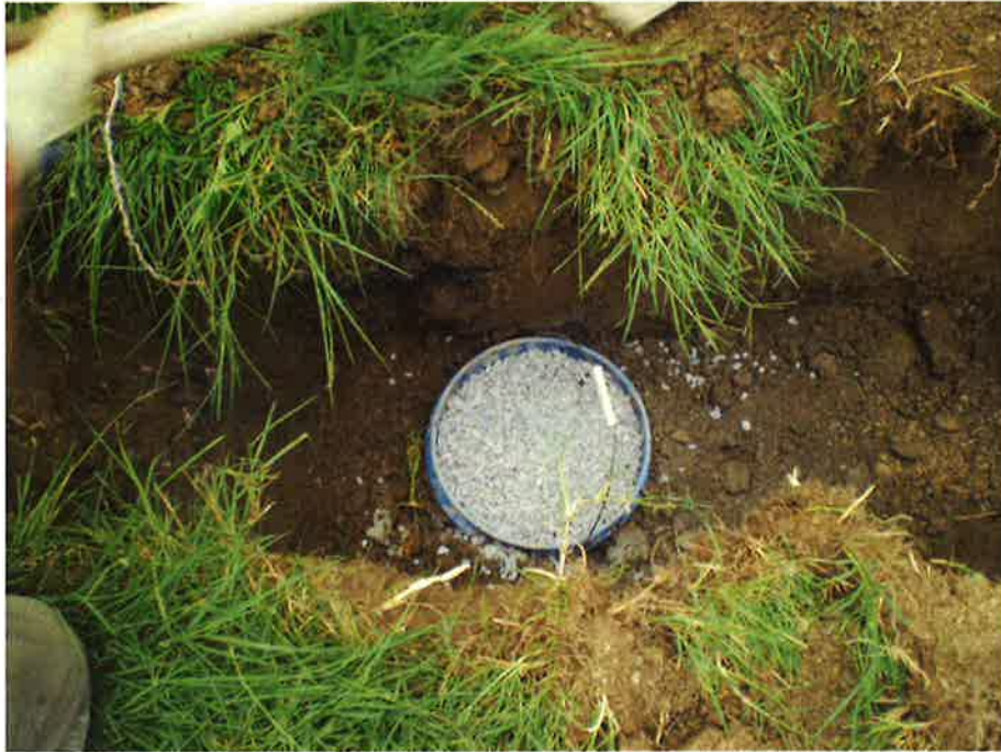
Photo 13. Placement of bentonite chips above MP-7G using a cut-off bucket as a form.
