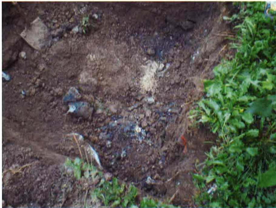
Photo 28. DPC and FPC excavated and cut off.
