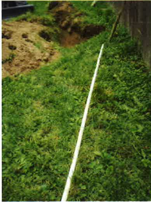
Photo 17. Probe casing pulled from MP-8G location.
