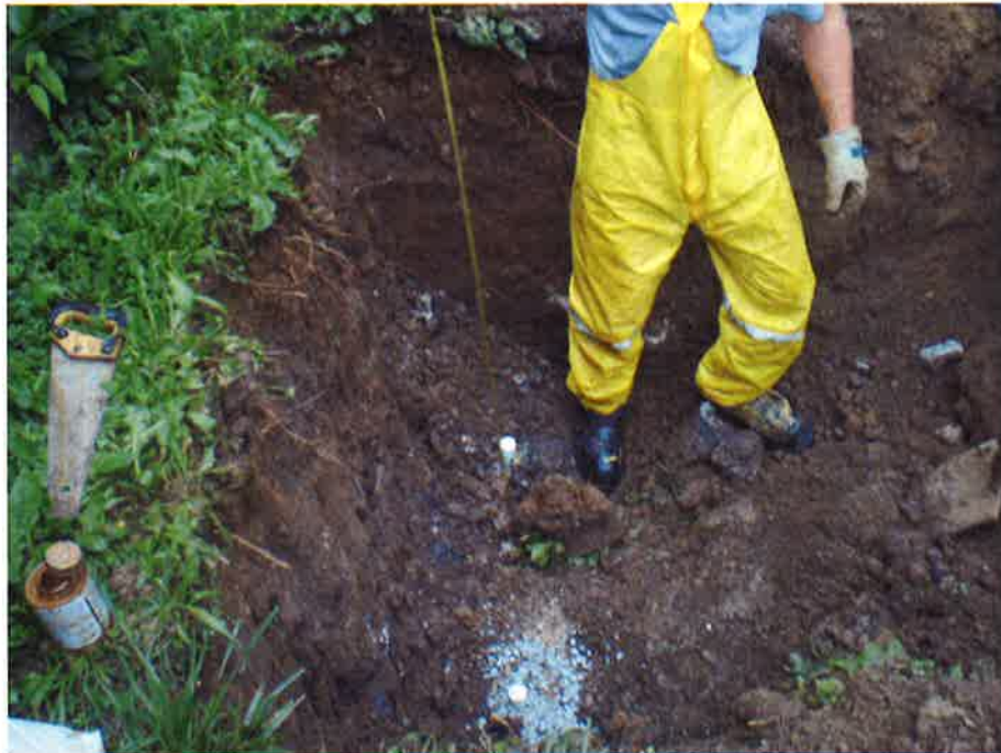
Photo 30. Checking depth of excavation at FPC.
