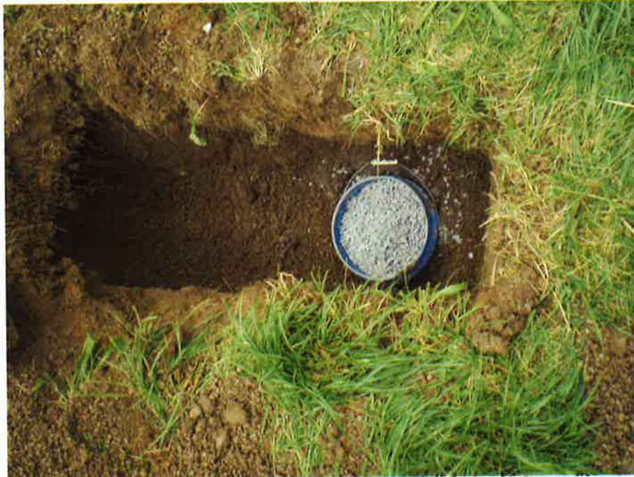
Photo 22. Bentonite placed in MP-8BR.
