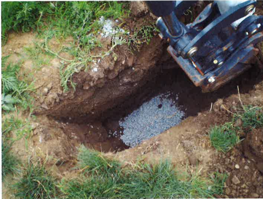
Photo 3. Bentonite chips placed in MP-15 excavation.
