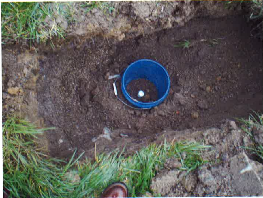
Photo 23. Bucket form placed above capped MP-8R and partially backfilled, prior to placement of bentonite chips.
