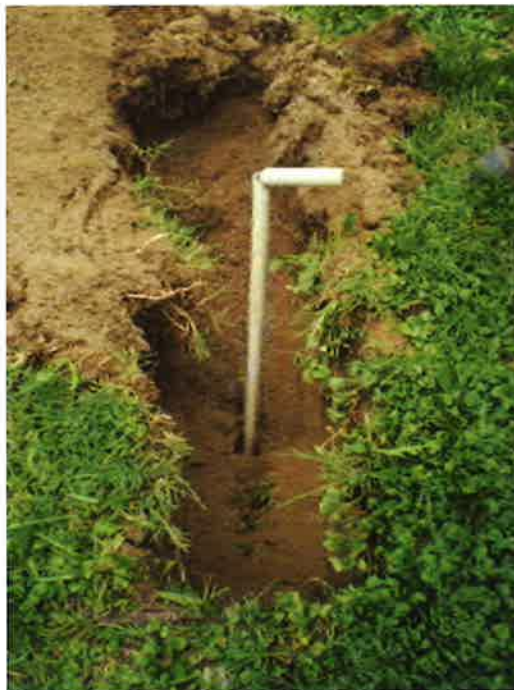
Photo 14. MP-8G casing pulled out of excavation.
