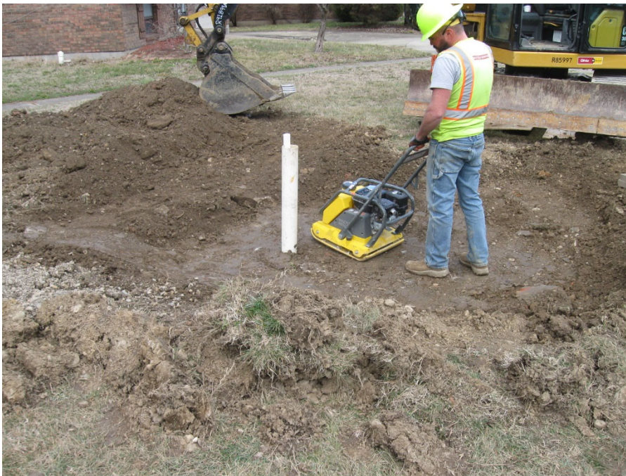
Photo 10: Vibrating plate compactor used to compact backfill.
