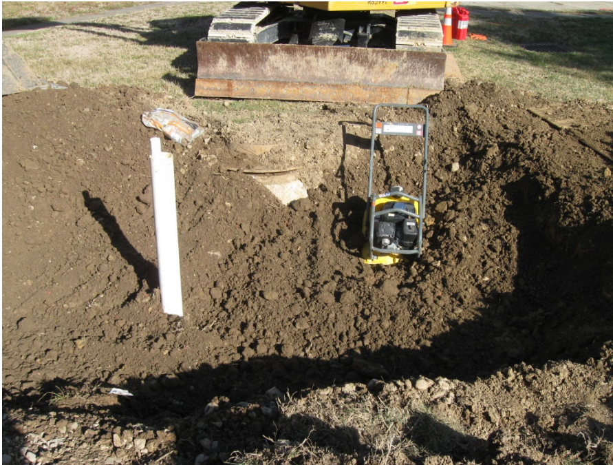
Photo 9: Vibrating plate compactor used to compact backfill.
