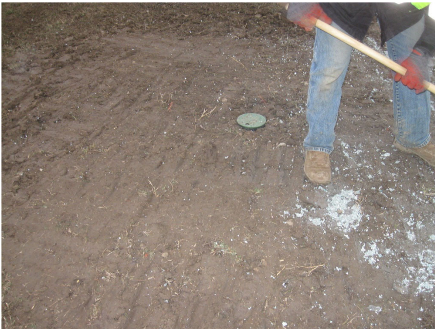
Photo 12: Completed valve box.
