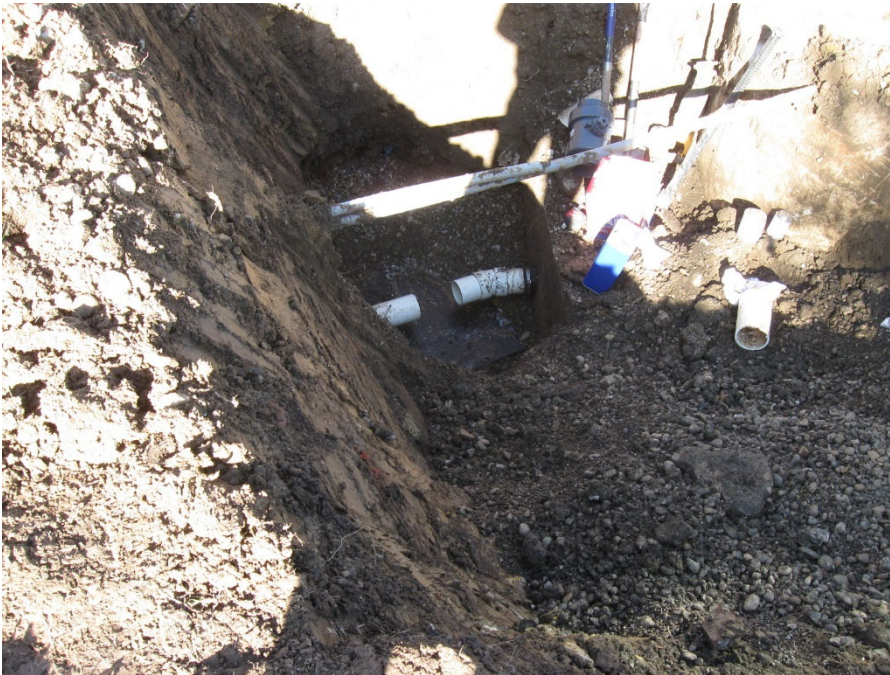
Photo 4: Condensate line cut and 24-inch square of HDPE placed below line.
