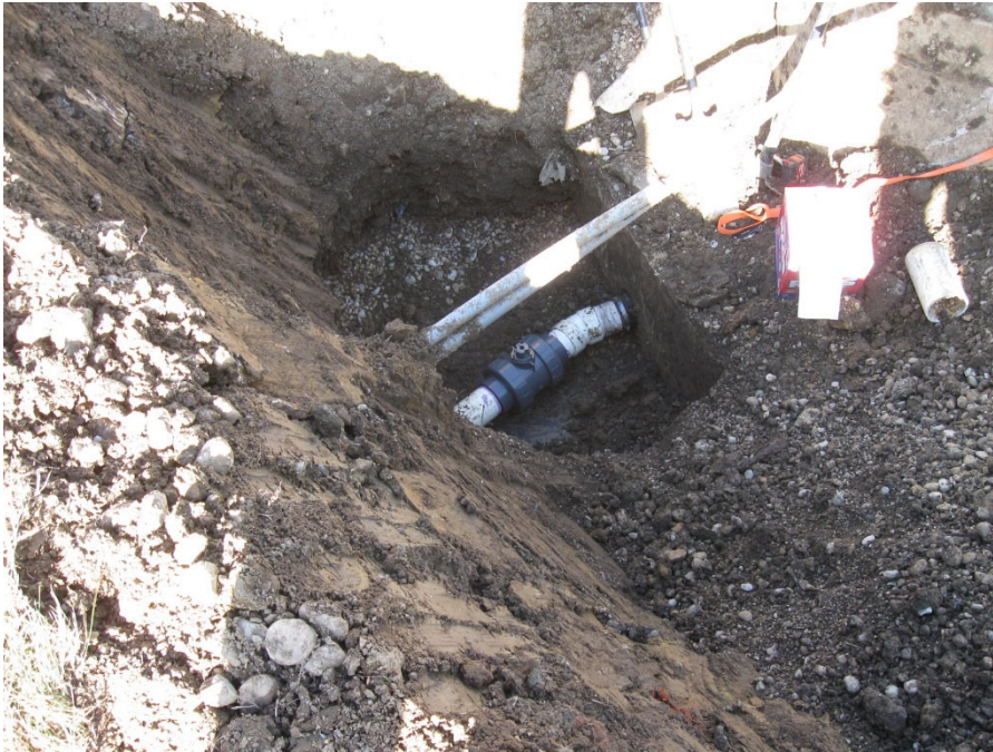
Photo 5: Valve installed.
