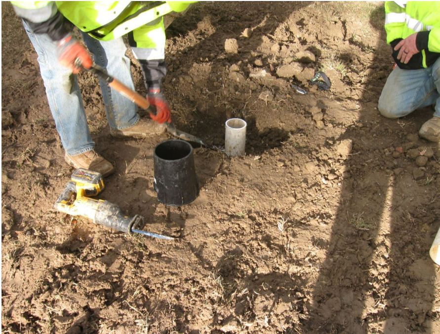
Photo 11: Preparing to place valve box.
