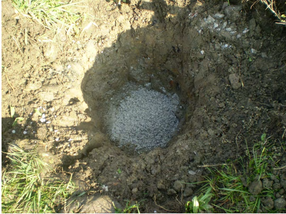
Photo 7. One foot of bentonite placed, prior to hydration.
