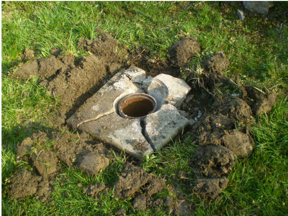
Photo 4. Concrete pad broken and in process of removal.
