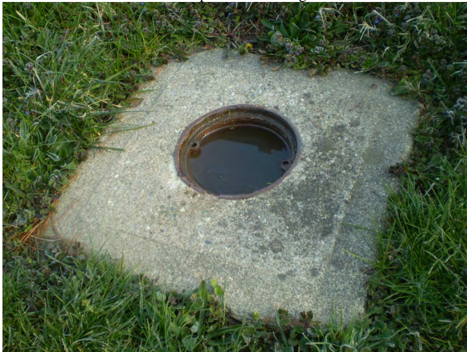
Photo 2. MP-10 with lid removed.
