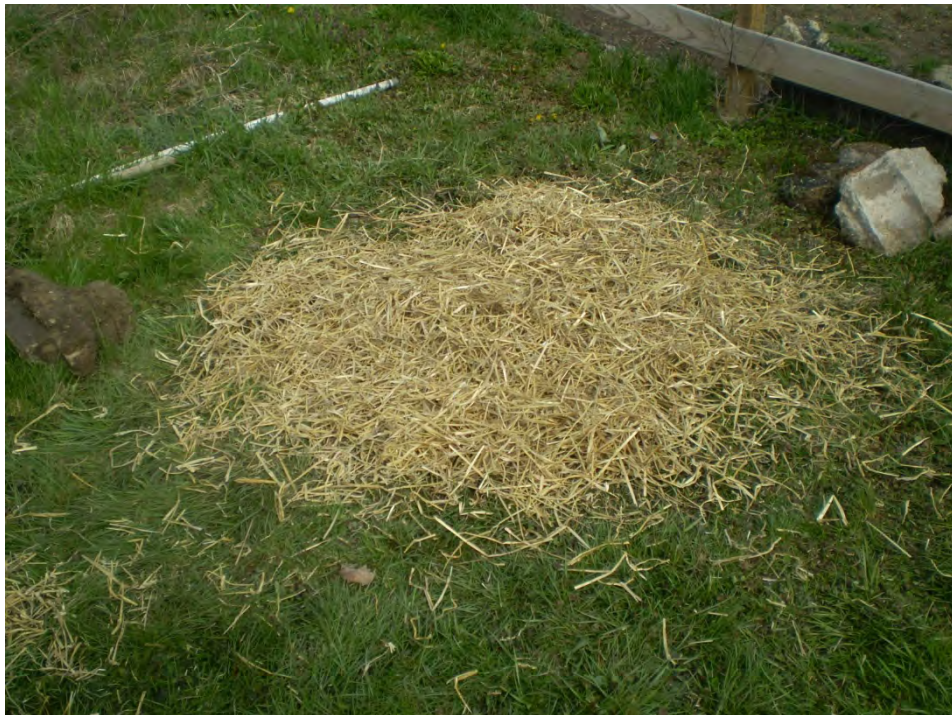
Photo 8. Backfill, seeding, and mulching completed.
