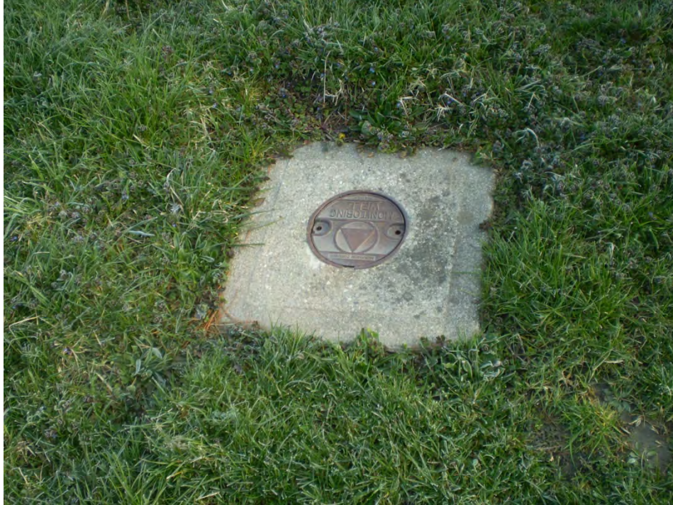
Photo 1. MP-10 flush mount protective casing.
